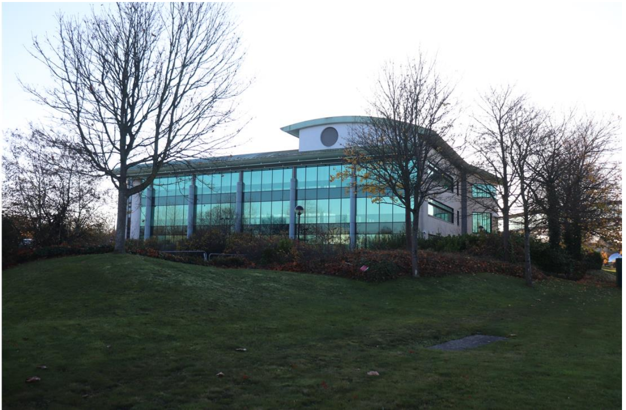
Application site from M3 Junction 3 (Building 1)
